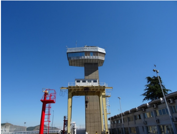
Figure 3.6 - Navigational lock "Djerdap I", command tower
