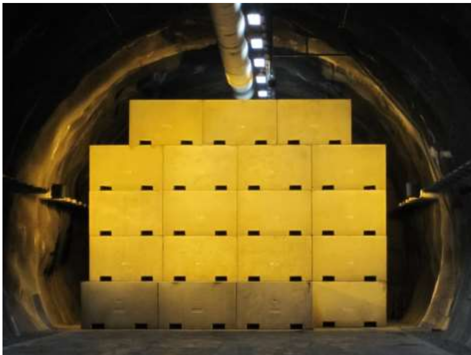
Figure 13: Placement of reinforced concrete containers in storage chamber I-K1 of the NRWDF
