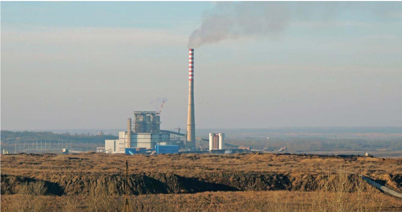
Figure 10. Mines and thermal power plants dominate the landscape – Kostolac thermal power plant and Drmno open cast mine. Photo: Milan Paunovic, original.
