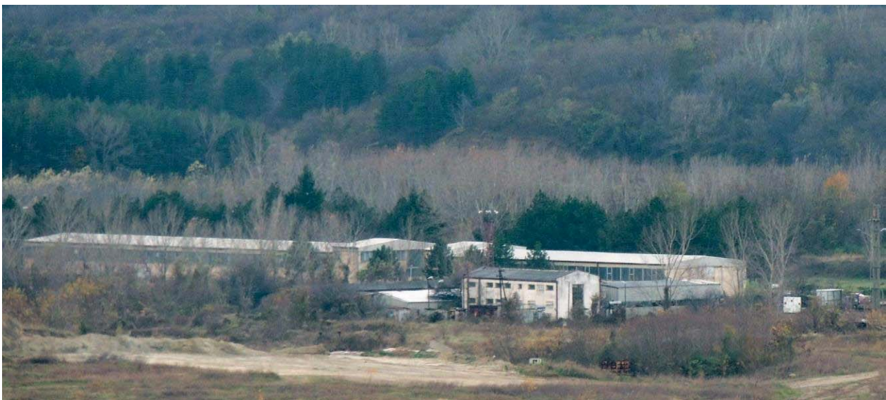
Figure 13. Part of the Cirikovac open cast mine management complex buildings. Photo: Milan Paunovic, original.
