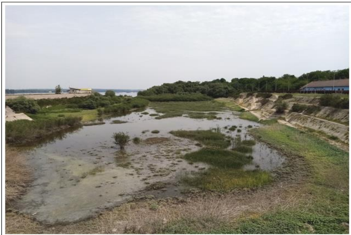
Picture No. 4: Port of Prahovo – „Zimovnik“ - existing condition
