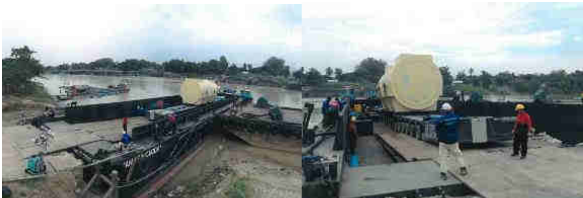
Figure 4.7. Pontoon bridge/barge with a stator load of about 400 tons
