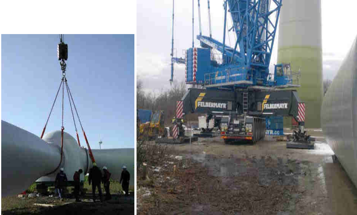
Figure 3.8. Photographs with an example of assembly of the blade parts
