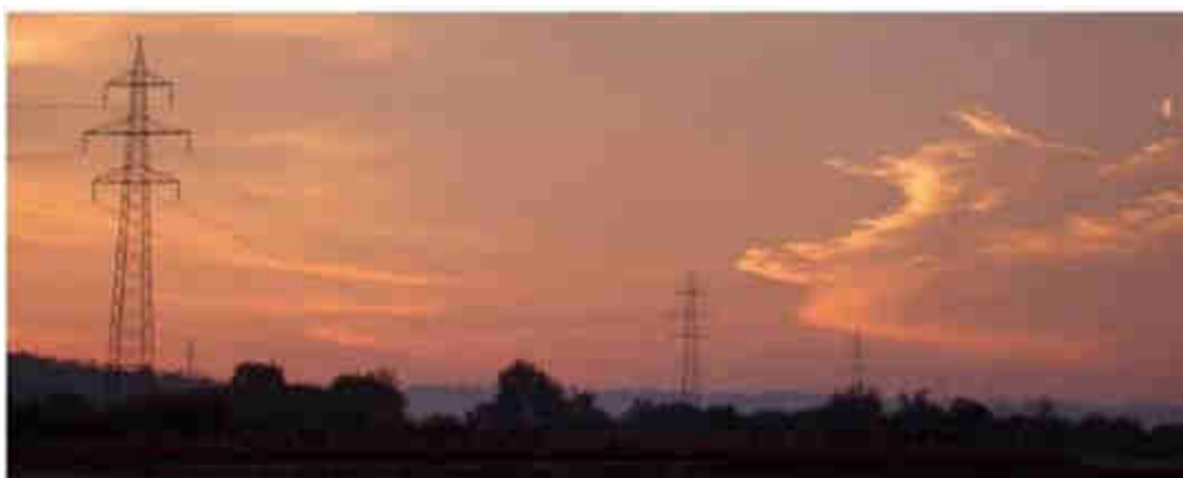
Figure 2.28. Several high-voltage power lines are located in the planned area
