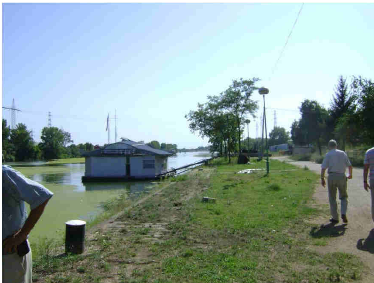
Figure 3.12. North side of the channel
