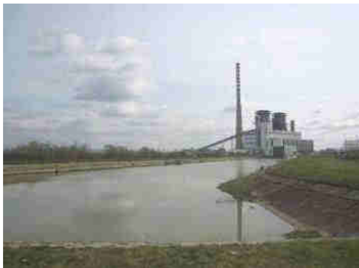
Figure 2.25. Cold water channel
