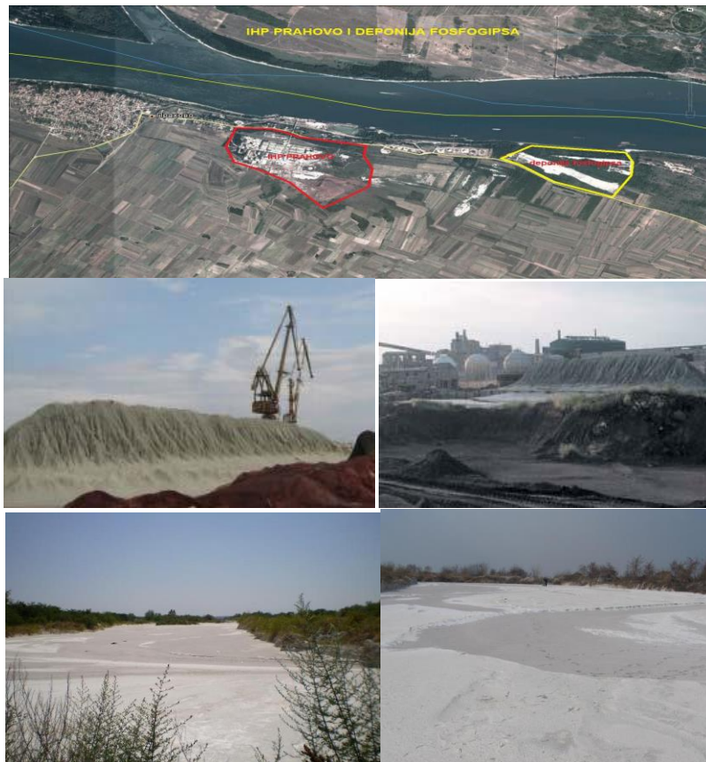
Fig.5.5 Location and view of the existing phosphogypsum storage IHP Prahovo
