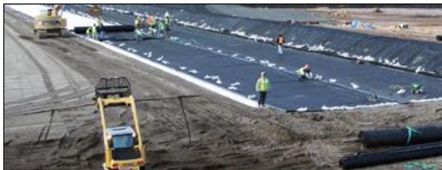
▪ Fig.8.1 Liner spreading along the storage cassette's bottom
