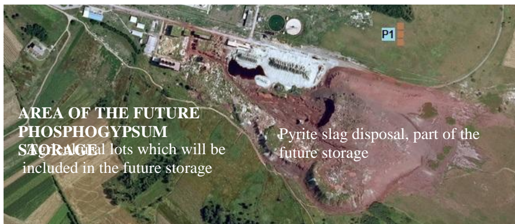
Fig.2.7 Location of piezometer (P1) in relation to the location of the future storage
