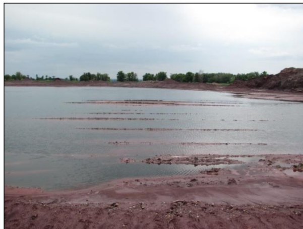
Figure 6.17: Pyrite slag disposal under water from precipitation
