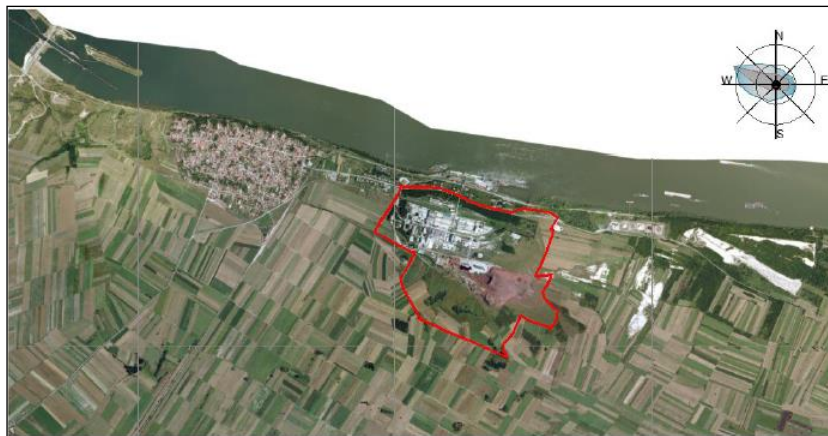
Fig.2.2 Satellite photo of the location of the complex Elixir Prahovo Ltd Prahovo
