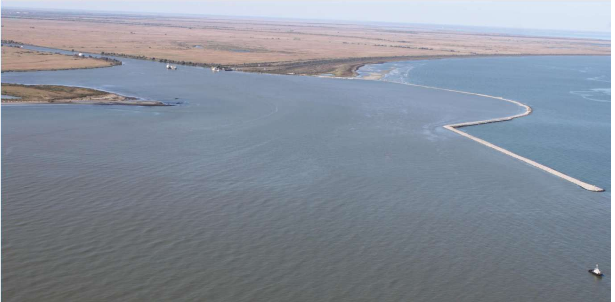
Figure 1.2 Bar section of Bystre arm (existing condition)
