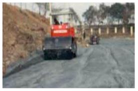
Figure 3.3.4-13: Vibrating roller working on compacting
