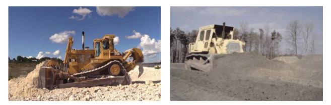
Figure 3.3.4-12: Bulldozers working on spreading and planning
