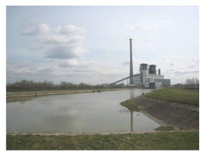
Figure 2.5-6: Cold water channel
